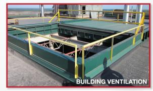
Two 18' x 18' Sliding Roof Hatches used for large equipment access and power plant ventilation. Manually operated.
