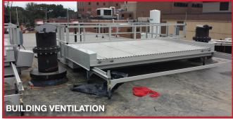
16' x 8' Sliding Roof Hatch used for hospital exhaust control/ventilation. Power operated.
