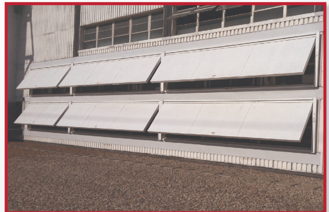
60' x 10' top pivot louvers used for building ventilation at a power station.
