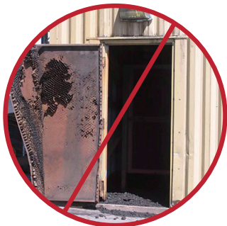
Failed Hollow Metal Door
