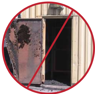
Failed Hollow Metal Door
